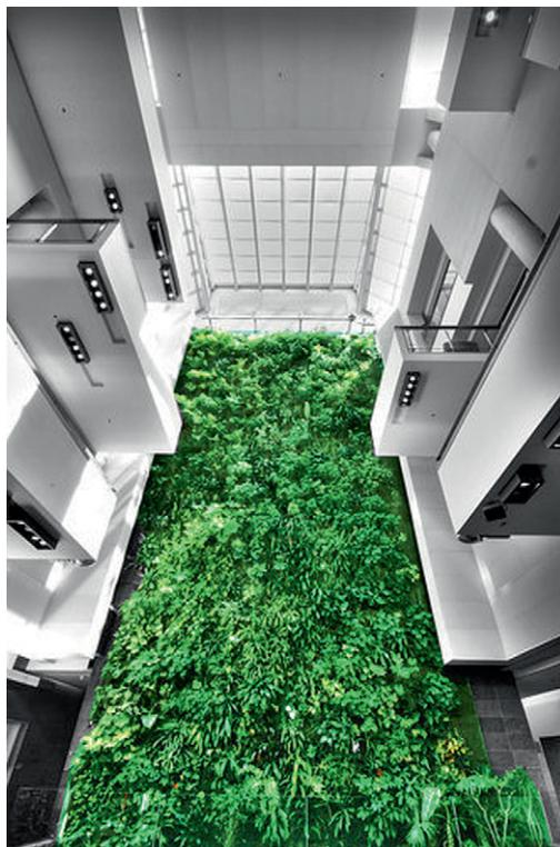
**Figure 2** Example of a typical botanical indoor air biofilter installation, located in the atrium of the University of Guelph-Humber building, Humber College, <http://www.guelphhumber.ca/>, photo courtesy of Nedlaw Living Walls Ltd.
